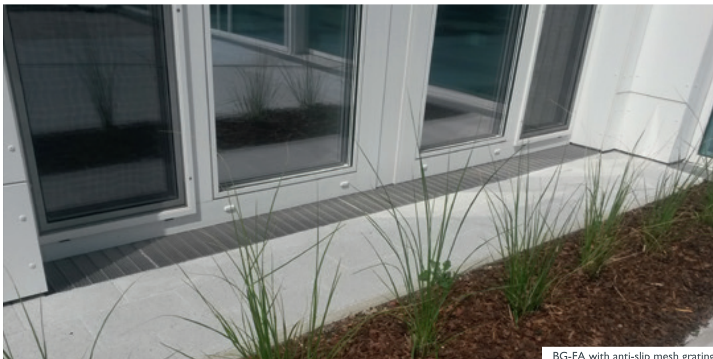
BG-FA with anti-slip mesh grating
